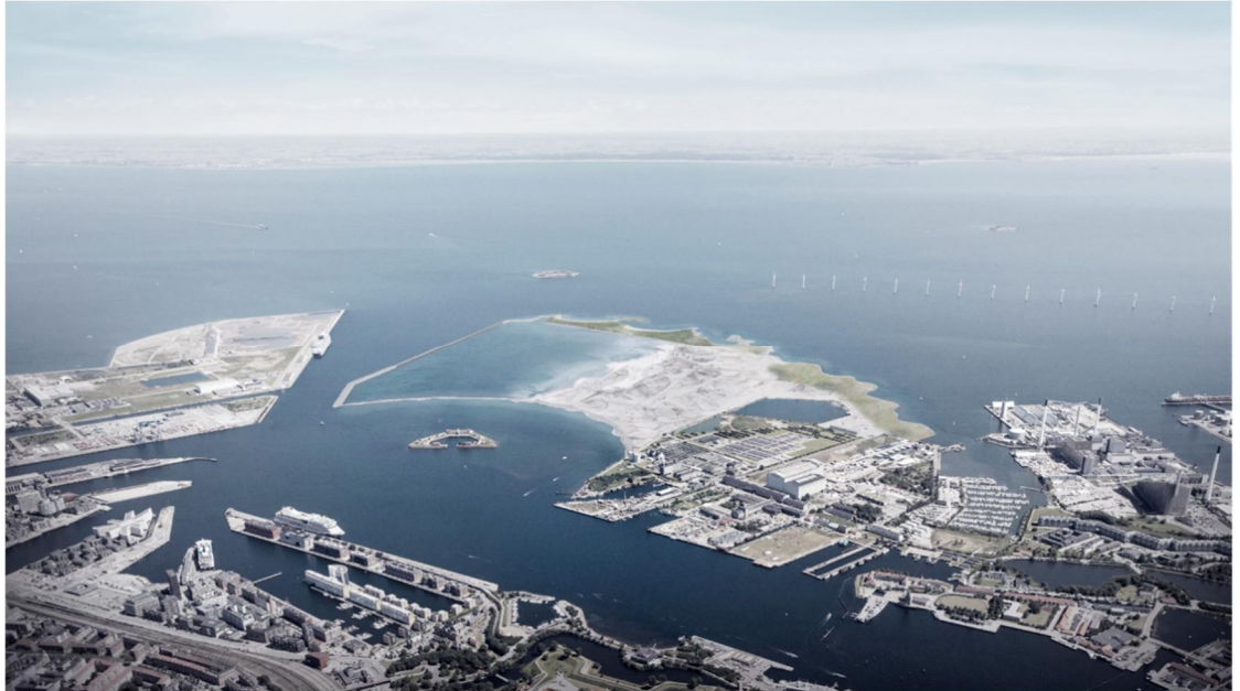
Figure 1.1 Artist impression of the Lynetteholm land reclamation in the center with Copenhagen in the foreground and the Øresund with the Swedish coast in the background (Source: By & Havn).
