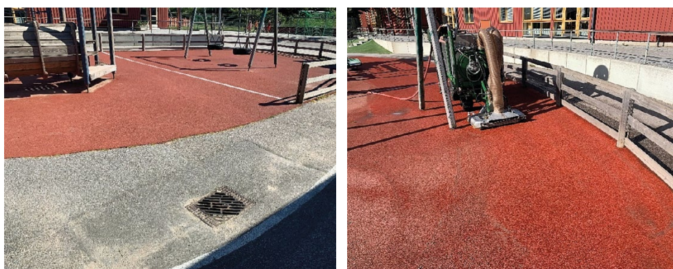
Figure 34. Photo taken before and during cleaning. Filter installed in drain.
