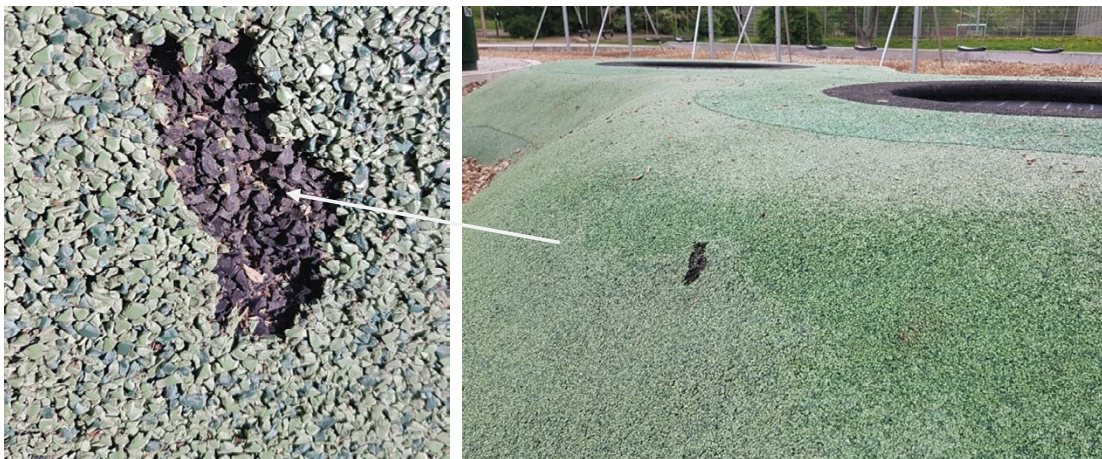
Figure 3. Fall safety surface where the top layer has been damaged and the base layer is exposed. Photo: Åsa Jarsèn.
