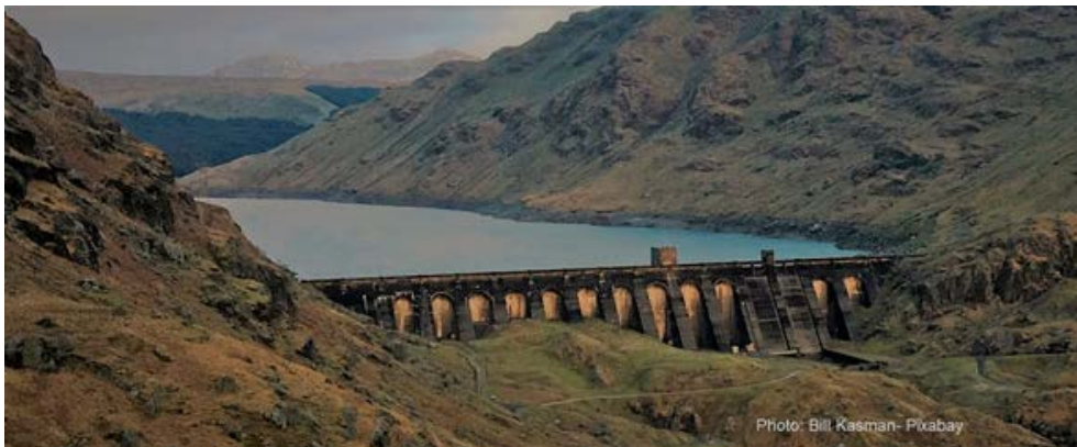
Figure 2.47. The dam is a beautiful engineering work, made to last over 100 years.
