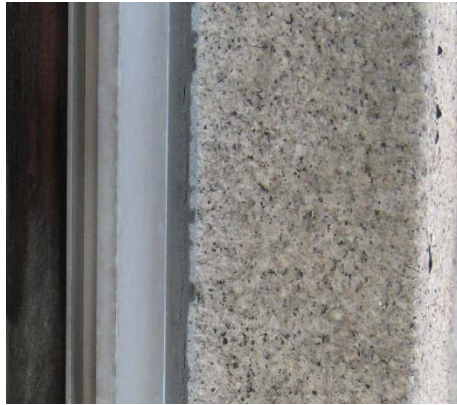
Sealant between a window and natural stone
