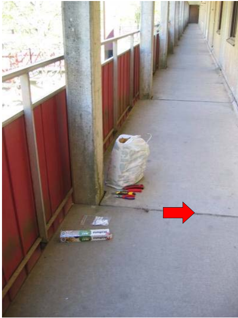
Sealant in exterior passageway
