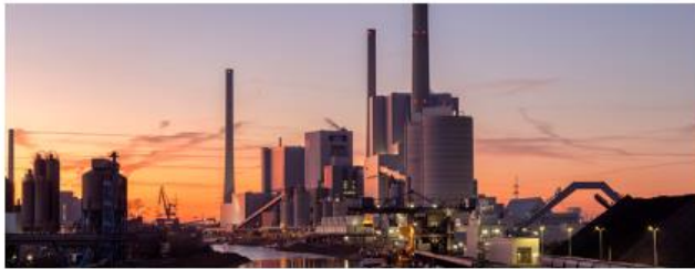
Power generation: Strengthen control over emissions from coal-fired power plants and increase penetration rates of new renewable energy
